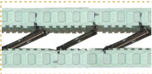
Close view of folding metal-hinged web
