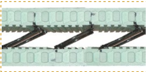
Close view of folding metal-hinged web
