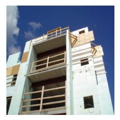
Window and Door openings are also prepared during build using permanent or temporary buck materials which will support concrete during placement. Once at projected wall height, vertical reinforcing steel is inserted into wall cavity as specified. Concrete placement is recommended using boom pump and internal vibration to assure even placement and monolithic pour condition.
