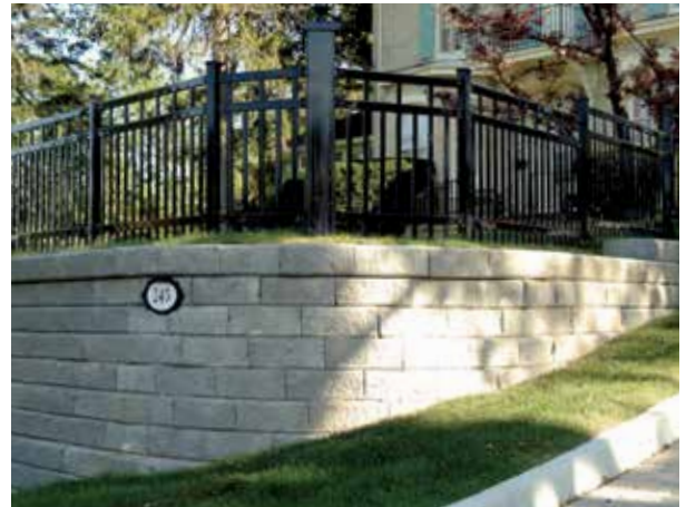
Grande walls allow for curved designs
