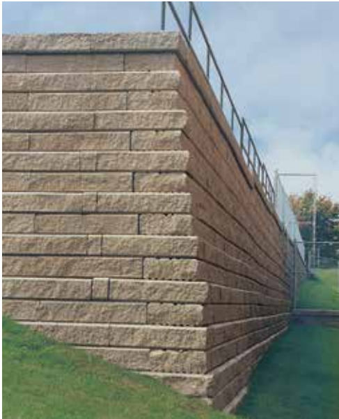
Using geogrid lets you increase wall height and minimize construction costs.
