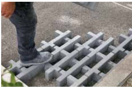
Boulevard Verde pavers are laid in strips on a conventional densified granular foundation.
