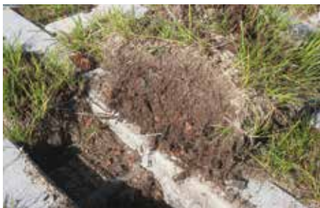
For grass pavements exposed to a lot of vehicle traffic, the recommended fill is structural soil.
