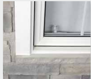
Finish with window sill, trim and jamb
